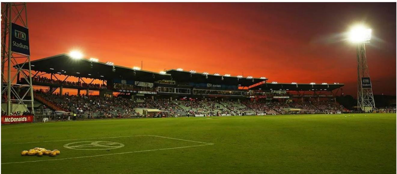
Figure 5: TIO Stadium in Darwin
