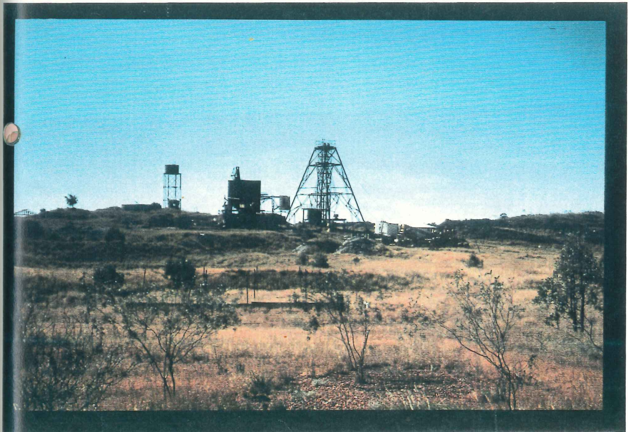
Remains of mining infrastructure Pioneer Complex, Hatches Creek
