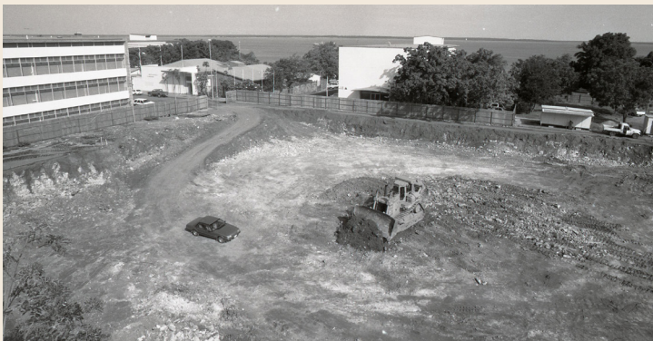
[Construction of State Square, foundation digging, 14 February 1989]
