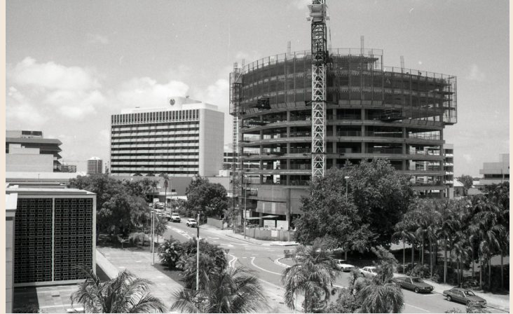
[Building construction, corner of Mitchell and Bennett Streets Darwin, 4 January 1989]
