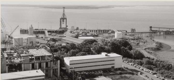
Darwin skyline from the roof on NT House [toward Fort Hill Wharf, Supreme Court under construction] 2 Feb 1990 LANT NTRS 3823 BW2881 Neg33
