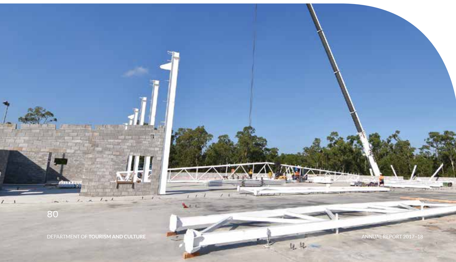
Construction of Darwin Indoor Netball Stadium.
